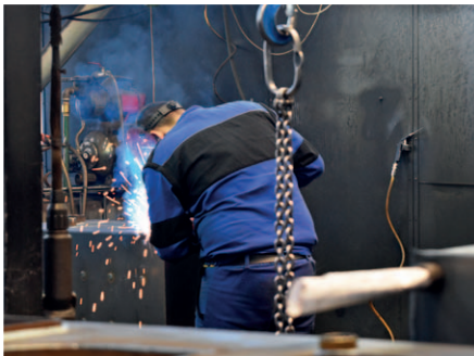
Manual boiler welding
